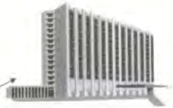
Acute care facility
